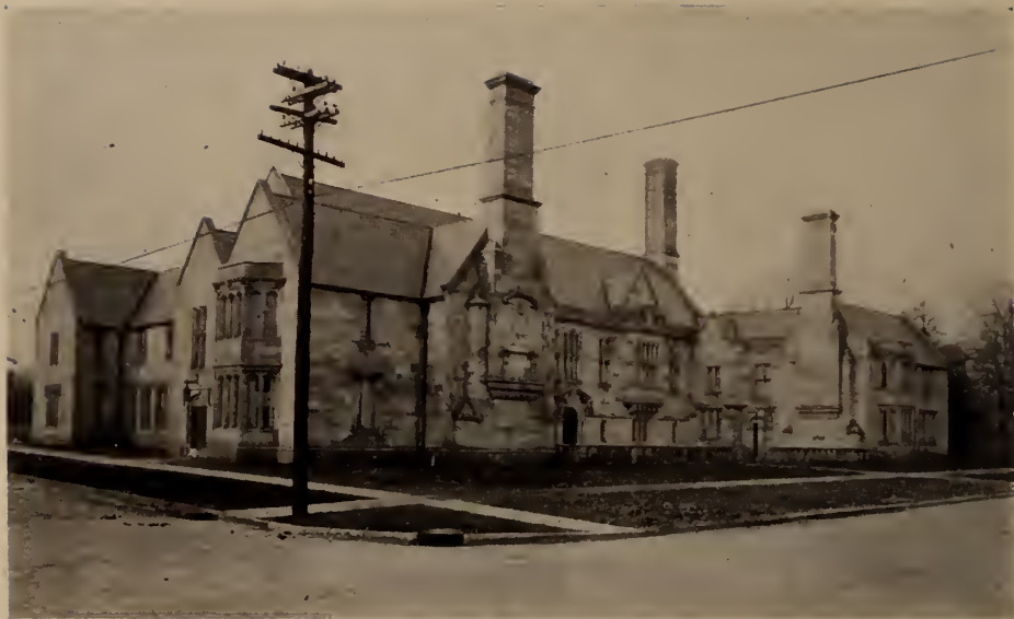
The Wesley Foundation, the social center of the Methodist Church. A church building far surpassing this in size is to be built next year to the right to cost $500,000
